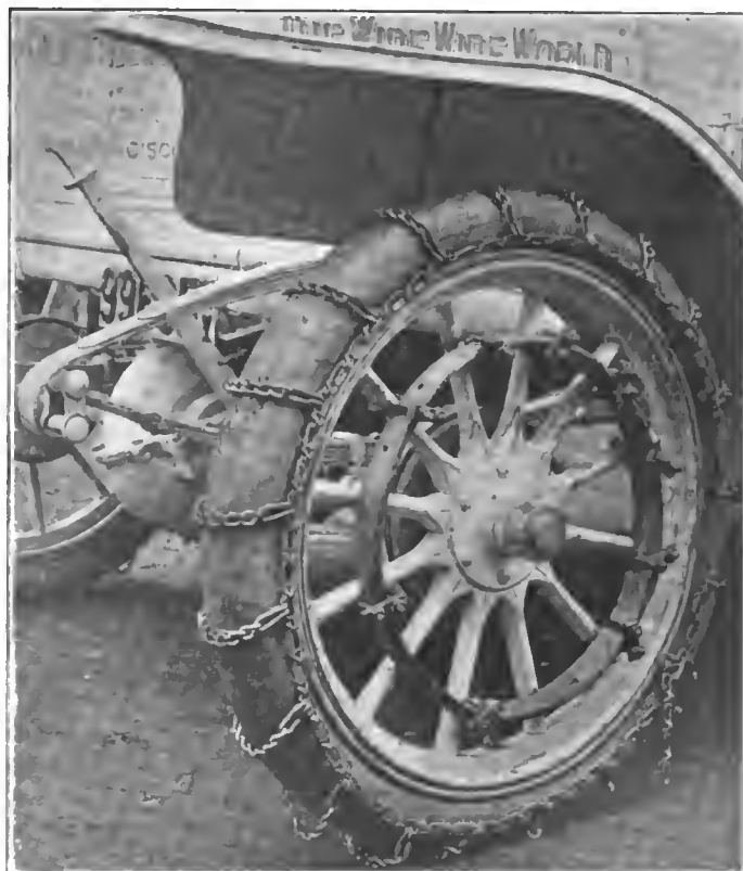
How the Overland's Battered Right Rear Wheel Was Stiffened
